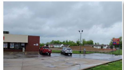
UDF at Wolfpen, with new construction in background
